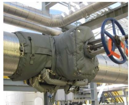
ThermoWrap blankets are generally used in lower temperature applications (typically well below 500°F) than their diesel and gas engine counterparts, where temperatures run 600°F and upwards.
