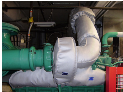
Pattern Designed, Blankets Installed
