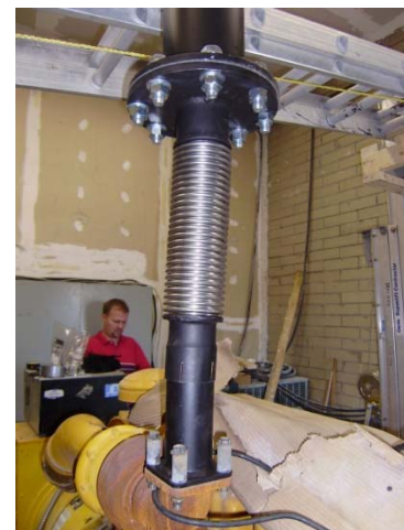
Firwin Engineer taking Measurements
