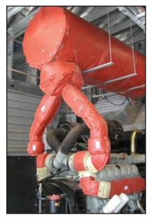
Blanket insulation is generally easier to install and also provides a higher degree of sound attenuation.
