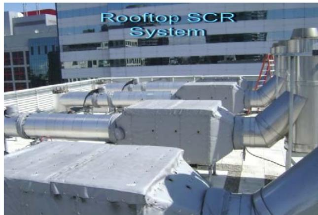
Firwin will also incorporate design modifications into blankets that are to be used for outdoor applications, such as extra flaps to reduce the amount of water that may get in underneath a blanket. Should the application be such where corrosion is known to be a potential issue, the company may recommend consulting with an outside corrosion engineer.
