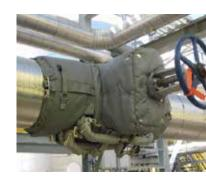
es, and are custom manufactured to precisely fit and easily install around a customer's valves, flanges, and engine and exhaust components.
