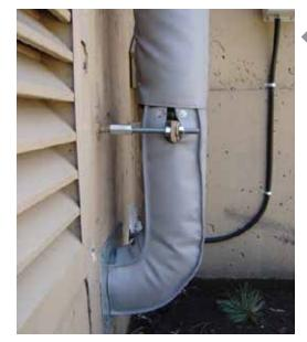
Removable insulation covers incorporate flaps, closures, and cutouts to provide easy access to ports and controls.
