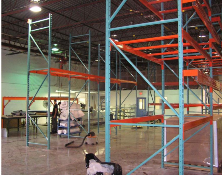
Floor Coated, New Storage Racks
