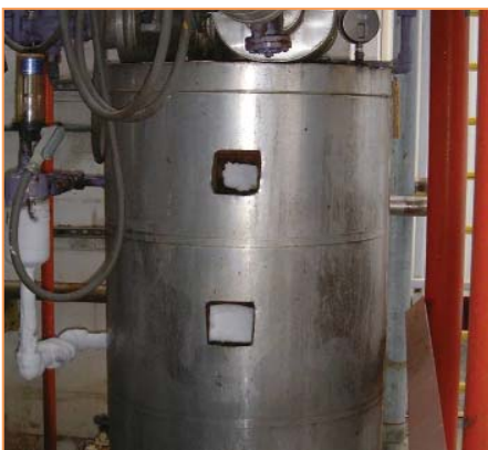
Figure 4: There are multiple inspection locations on this cold vessel.
