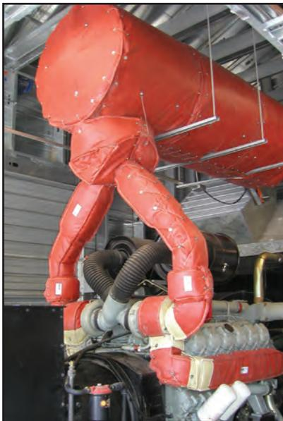
**Blanket insulation is generally easier to install and also provides a higher degree of sound attenuation.**
