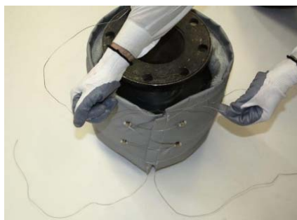
Installing Standard Firwin Flange Cover
